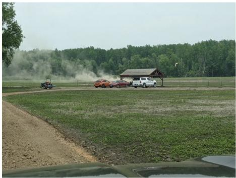
The accumulated silt on the runways is converted to dust as the power sweeper does its job. (Photo by Bob Breisemeister)
