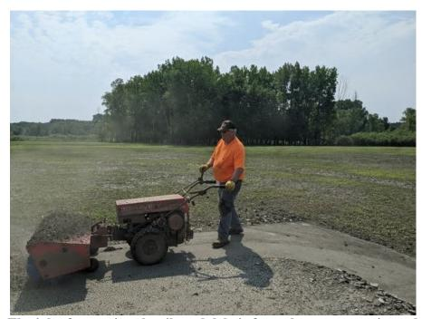
The job of removing the silt and debris from the runways, pits and taxiways would have been a lot harder without the power sweeper.
