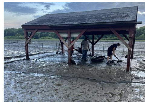
Trying to remove the silt from the shelter.
