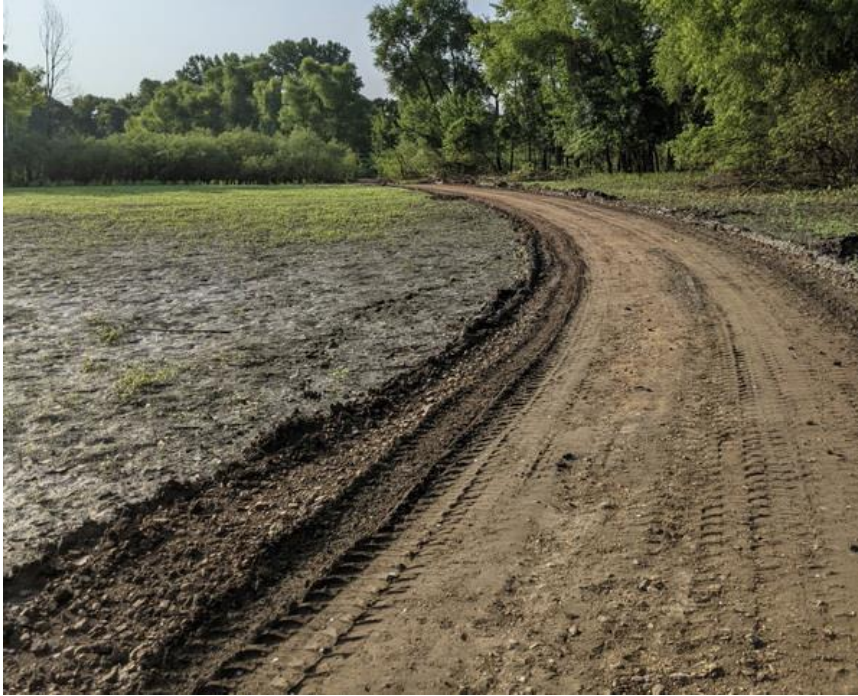
TCRC’s road to the field with the silt removed and newly graded. (Photos by Bob Breisemeister)
