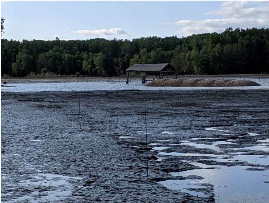
The water's almost gone, but now we must remove the silt and debris. (Photo by Bob Briesemeister)
